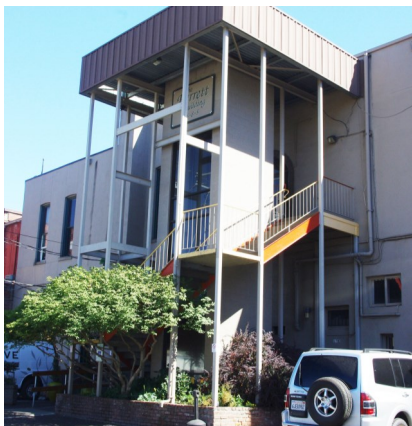
Combined Exterior Elevator & Emergency Egress
